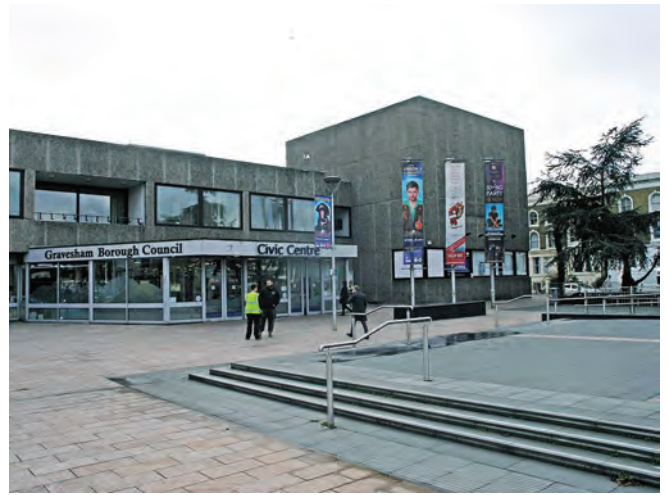
A new control centre at Woodville Halls, Gravesend, was under the block to the right
